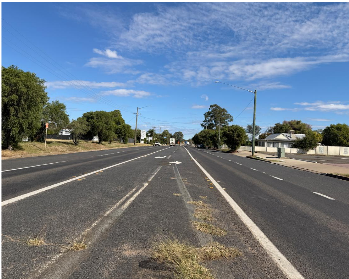
Looking south on Newell Highway/Cooma Road along site frontage
